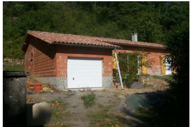
Typical brick dwelling. Bricks are usually rendered with plaster to improve water proofing
