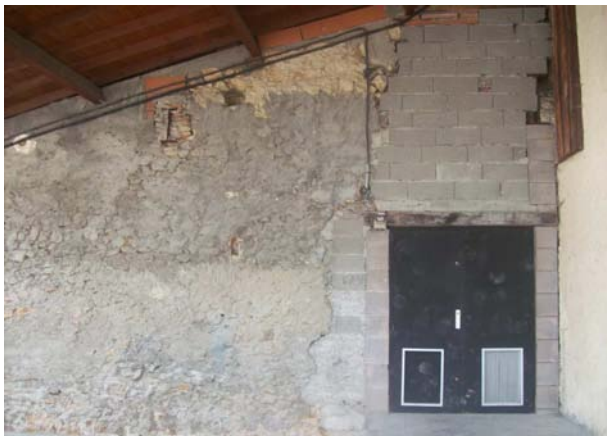
New fire exit added to local village music venue. Exit onto steps.
