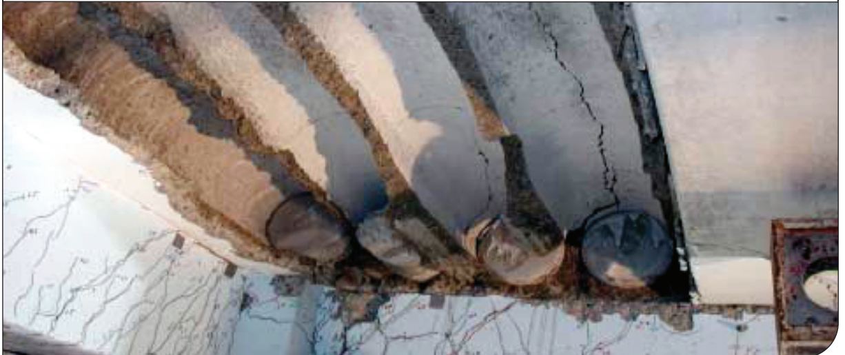
Figure 1 Example of failure in hollow-core flooring test after severe lateral displacement. Source: University of Canterbury, Department of Civil Engineering
