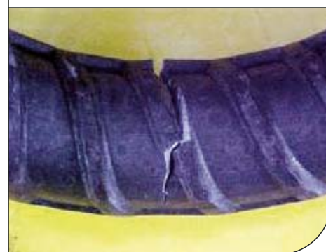
Figure 2 Cracks in Grade 500 reinforcement caused by incorrect bending and rebending
