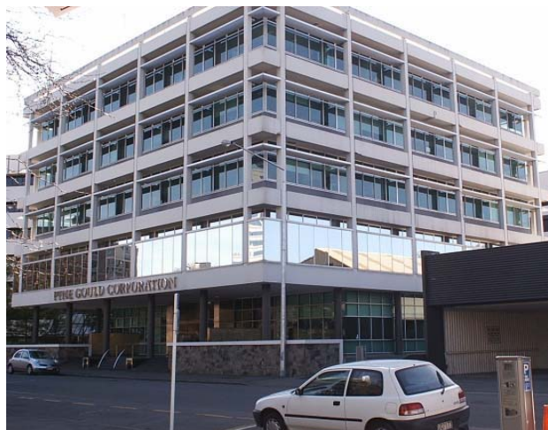
Figure 1: PGC Building prior to collapse (source: S. Tasligedik)
