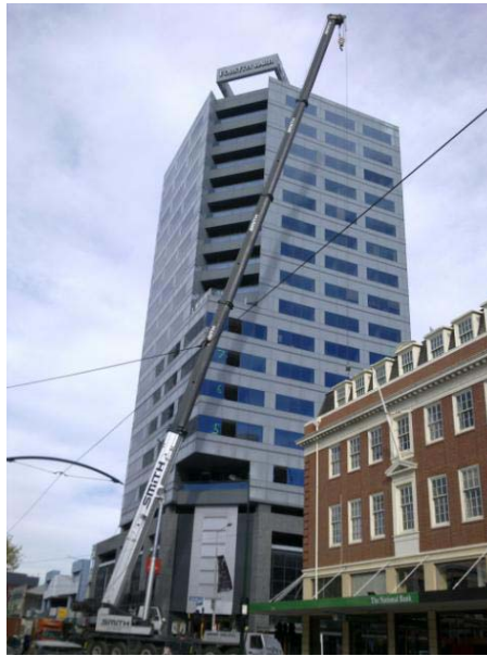
Figure 1: The Forsyth Barr Building from Armagh Street (looking south-east)
